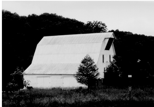
View of the east and north sides of the White Barn (2000). The shiplap siding and east-side doors were added in the 1930s. Note the large hay bonnet on the north.
