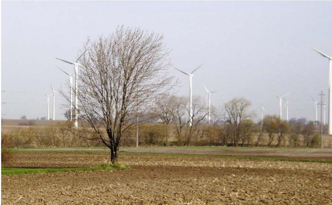
*Figure 8. The 800 kW turbines at Mendota Hills are the smallest size generally used in a utility-scale project.
