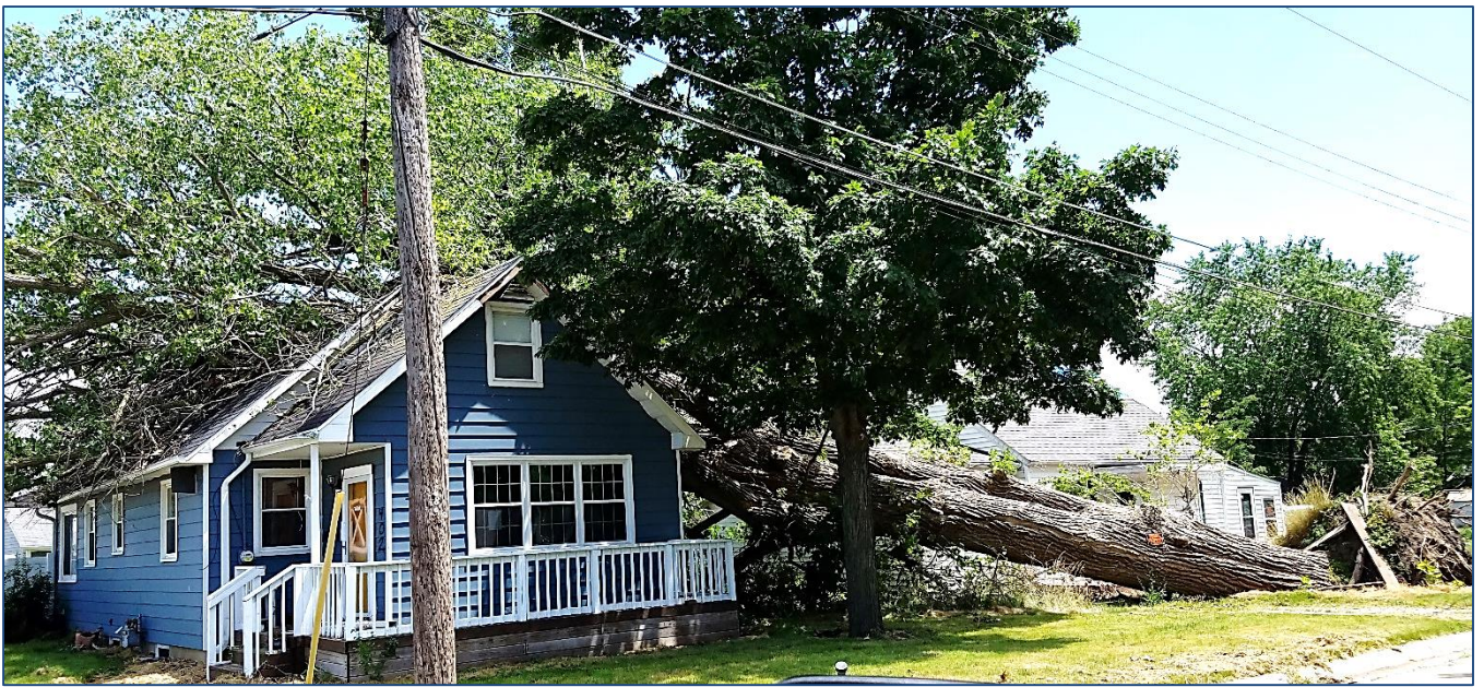
Severely damaged house from a large tree that fell from the February 28 th tornado.
