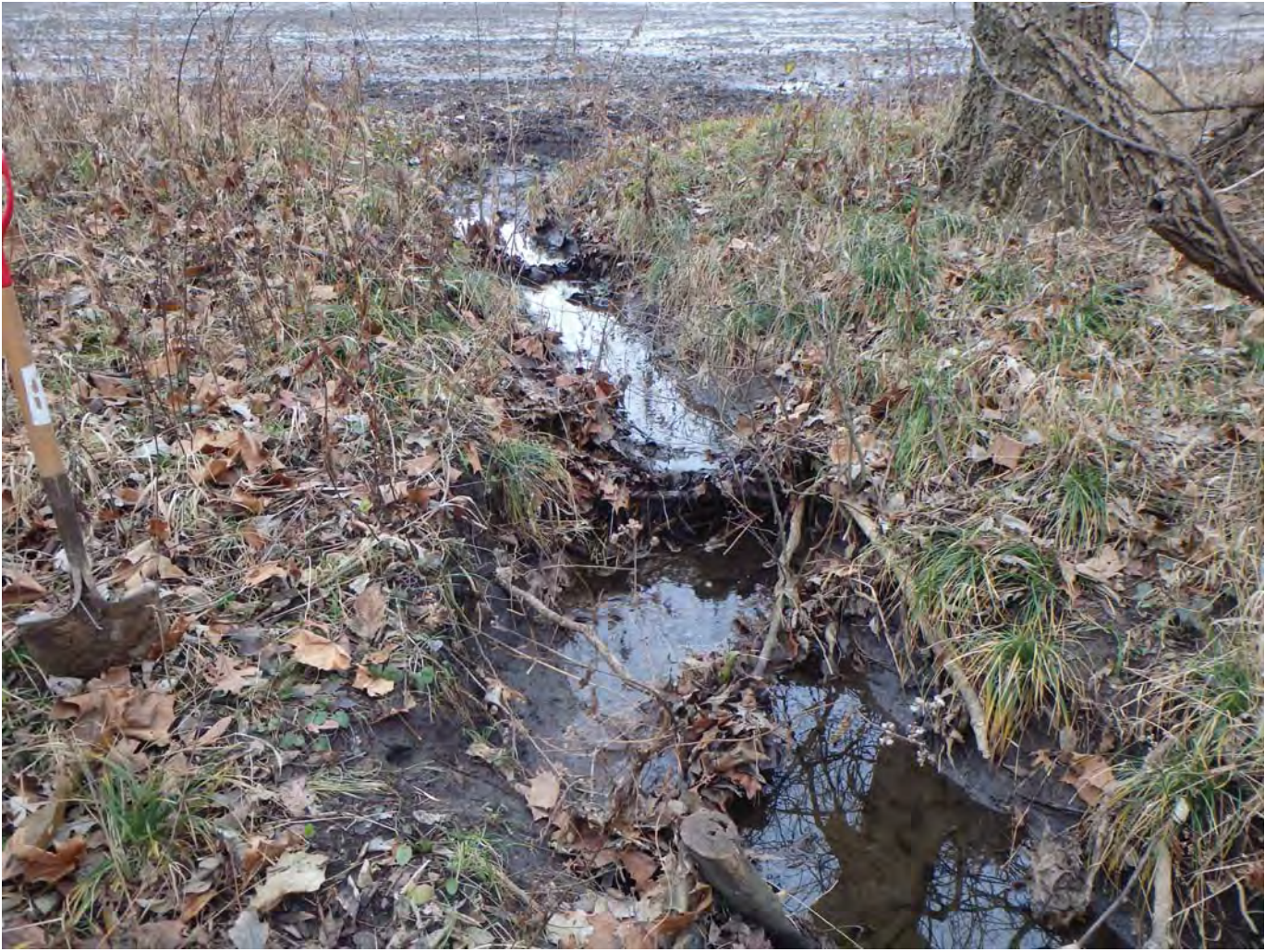
S6 looking upstream
