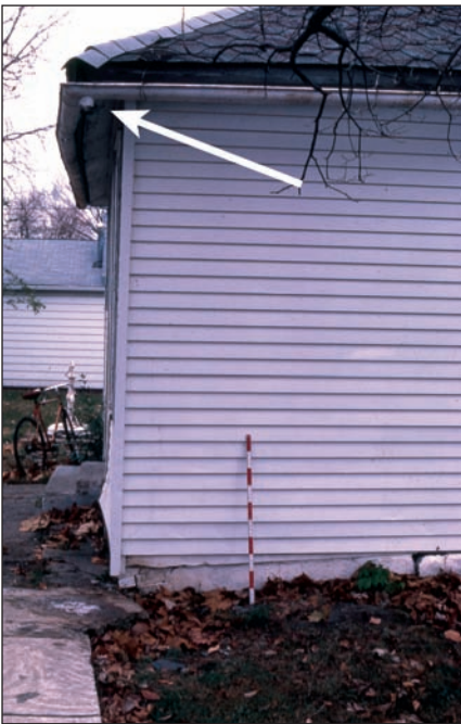
Figure 20 Foundation sinking at the corner of a building due to reduced support caused by excessive, repeated moisture changes. Note gutter drainage (arrow) and lack of downspout to channel drainage away from the foundation.
