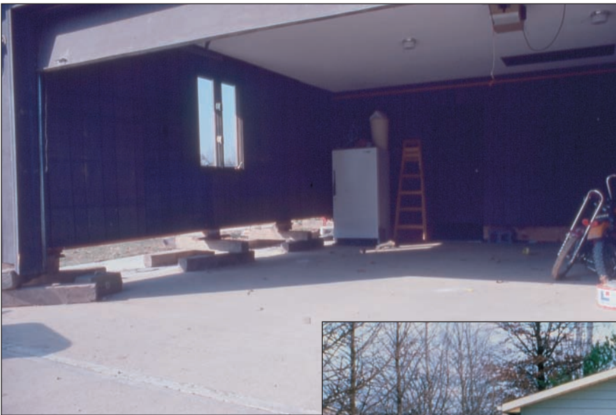
Figure 16 Load-bearing walls of a garage on a slab. The entire superstructure (frame) has been raised to a level position, exposing the interior of the garage. This re-leveling eliminates damaging stresses from differential movements of the foundation and maintains the superstructure level throughout the life of the event.
