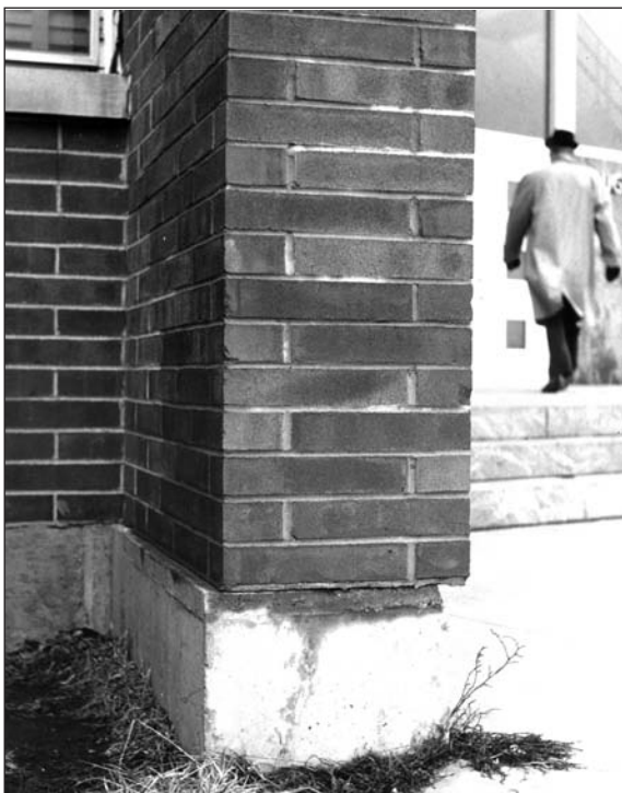
Figure 28 The largest movements are at the edges of the long, continuous wall. At this point, the short brick wall is being pushed off the foundation by the long, continuous brick wall to the left.
