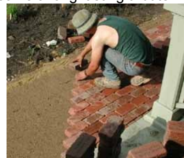
Dedicated Save the Prairie Volunteer building the walkway with your bricks
