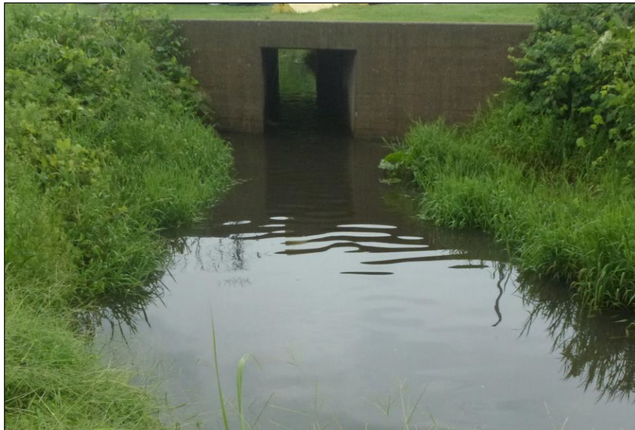
EXHIBIT 7 DEAD CREEK CS- F ( LOOKING EAST; 7 AUGUST 2018 )
