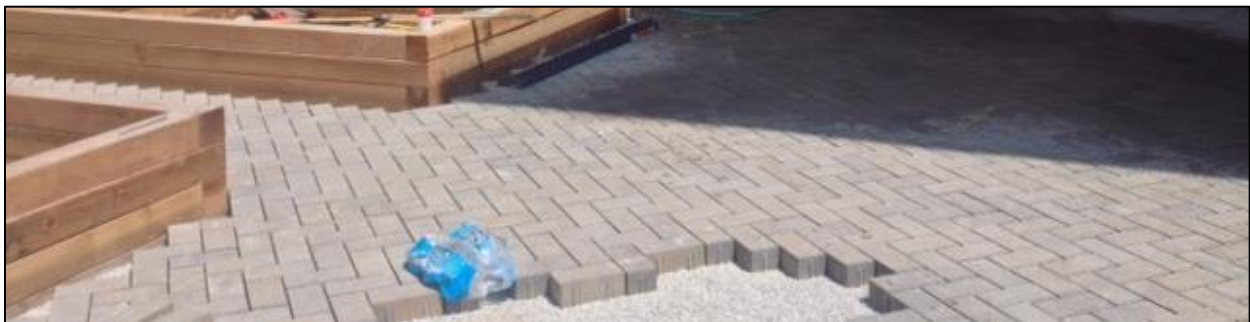
Permeable pavement during construction.
