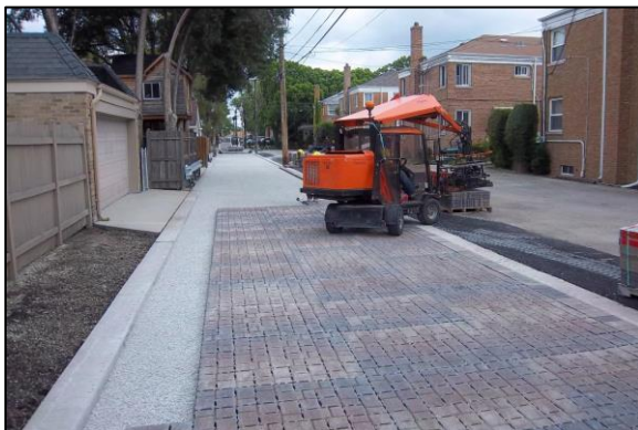
Permeable pavement alley during construction.
