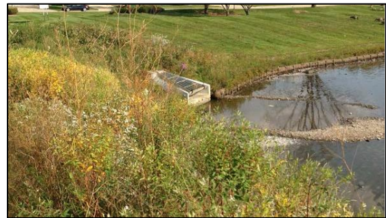
Shoreline buffer of native vegetation post-construction.
