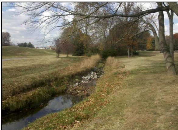
Two-stage ditch pre-construction.
