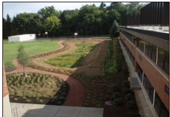
Rain garden post-construction.
