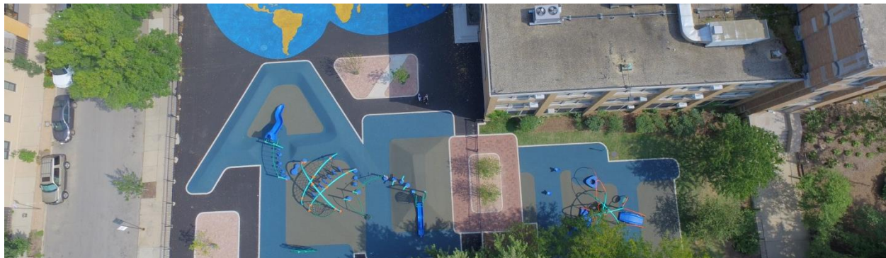
Permeable playground post-construction.
