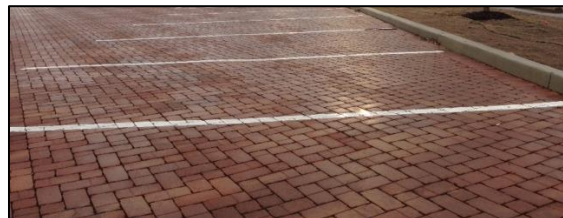
Permeable pavement parking lot post-construction.
