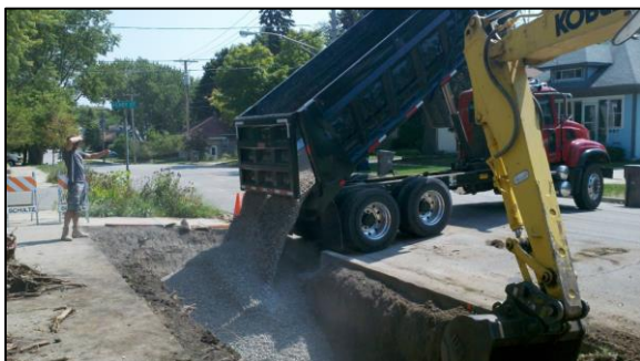
Bio-retention facility during construction.
