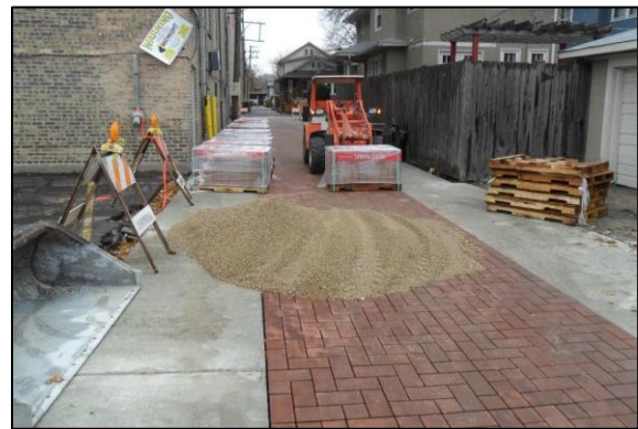
Permeable pavement alley during construction.
