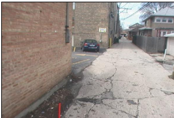
Permeable pavement alley pre-construction.
