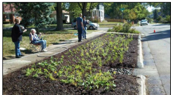
Bio-retention facility post-construction.
