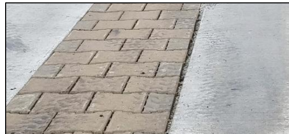
Permeable pavement alley post-construction.
