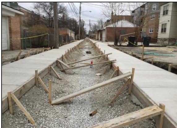
Permeable pavement alley during construction.
