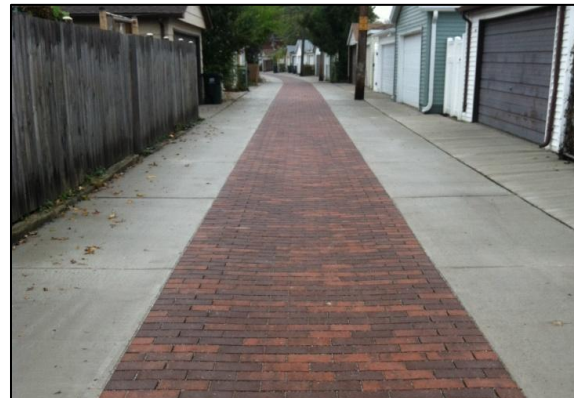
Permeable pavement alley post-construction.
