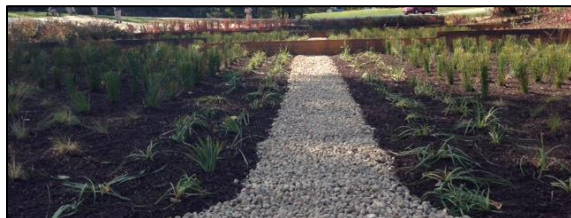
Bioswale post construction. 14-12(IGIG) SR
