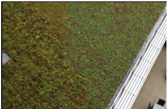
Green roof post-construction.
