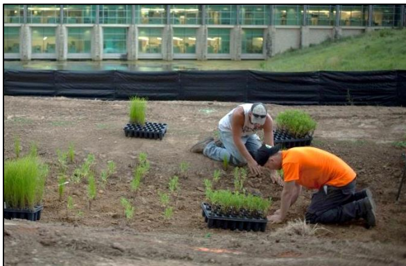
Bioswale during construction.
