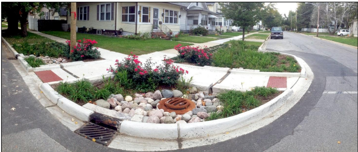
Rain garden post-construction.
