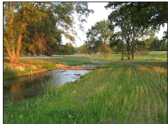
Two-stage ditch post-construction.
