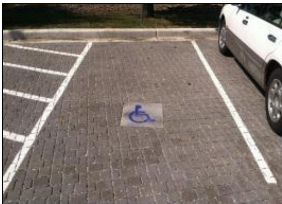
Permeable pavement parking lot post-construction.
