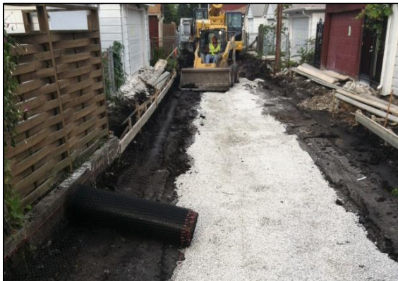
Permeable pavement alley during construction.
