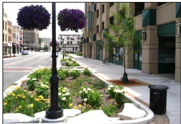
Bioinfiltration basins post construction.
