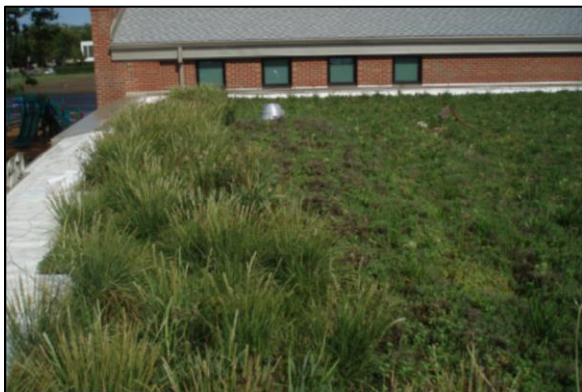
Green roof post-construction.
