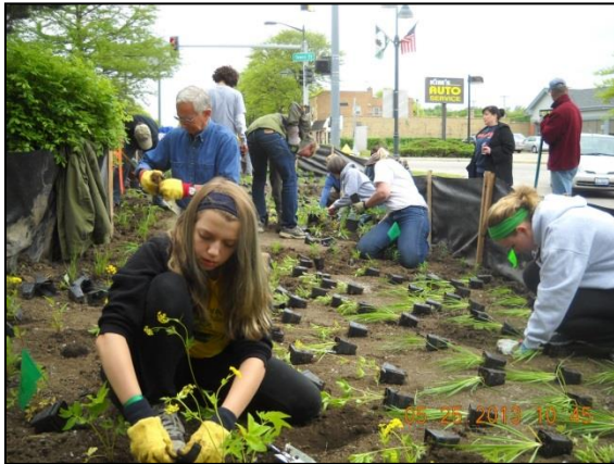
Rain garden during construction.
