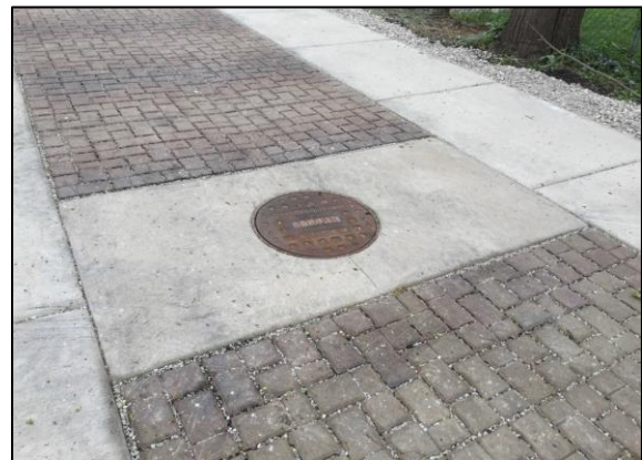
Permeable pavement alley post-construction.
