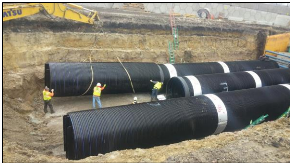
Water reuse cistern system during construction. 13-01(IGIG) JC
