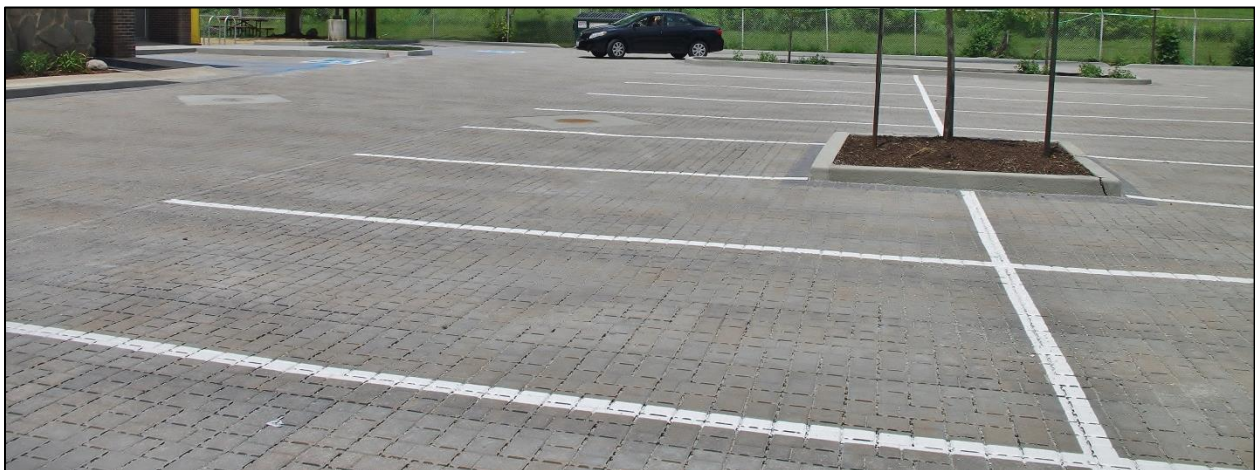
Permeable pavement parking lot post-construction.
