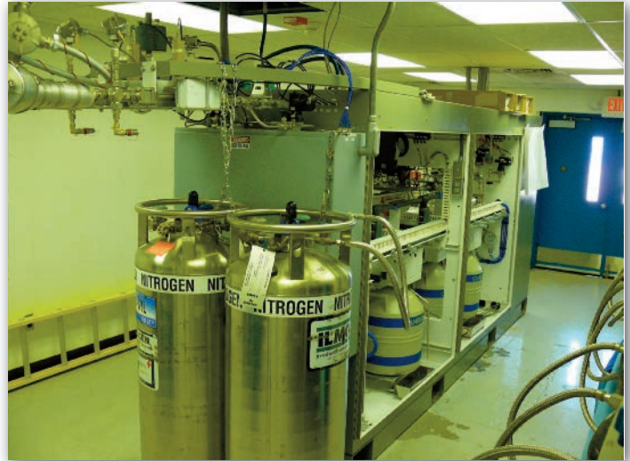
The GEMS measures and identifies radionuclides in each nuclear plant's effluent stack.
