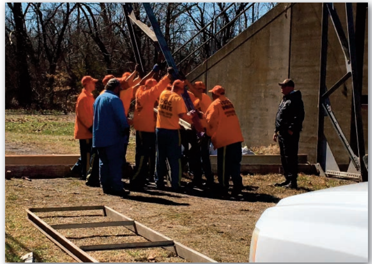
Inmates from the Illinois Department of Corrections Dixon Springs Impact Incarceration Program assisted with installing a floodwall along the Ohio River in Hardin County.
